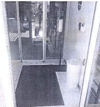
Figure 8 - Disinfection barrier, entrance (admin. building)
